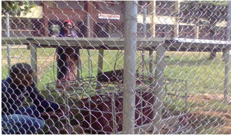
Fig. 1: The cubicle housing the PV system
