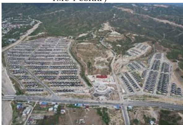
Figure 2. Residential Infrastructure Development Project in the Tondo 2 Area, Palu City (Source: TMC-1 CSRRP)
