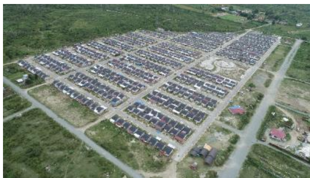
Figure 1. Residential Infrastructure Development Project I (Source: TMC-1 CSRRP)
