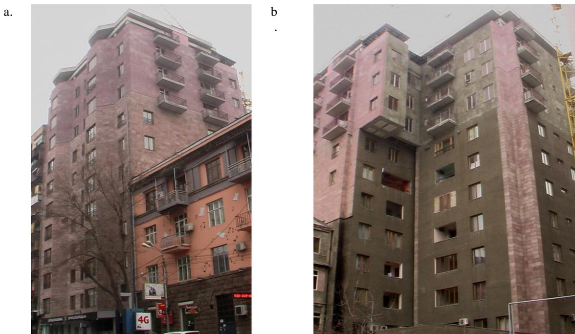
Figure 3. View of the existing 8-story building on Amiryan Street in Yerevan with the added four floors and a cover slab constructed on top and connected to the building by seismic isolators to form a dynamic vibration damper
